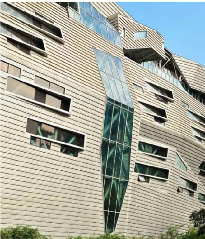
↑ The western facade is clad with seamless corrugated aluminium, punctured by small shaded fenestrations. These project towards the south to cut the glare, and are raked back on the northern side to maximise exposure to the cool northern light.
