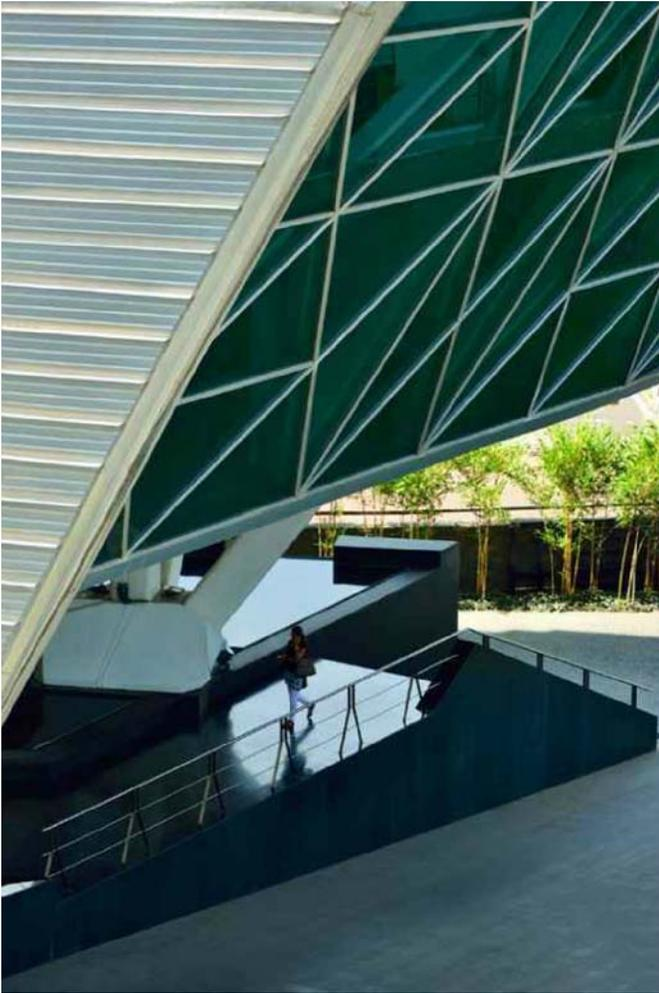
↑ The northern facade which receives the most light is angled back on the upper levels allowing maximum penetration of natural light through the laminated glass.
